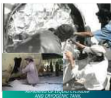
REFURBISHING OF EQUIPMENT FOR CRYOGENIC TANK
